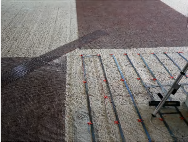
Carbon scrims on bare concrete slabs, with anode strips surrounding the supports to protect against cathodic corrosion (on the right)
