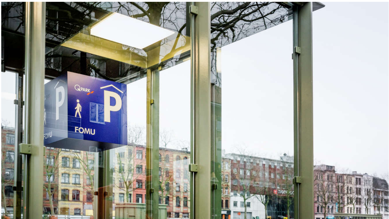
Figure 5: Pedestrian access/exit point near FOMU (Foto Museum)
